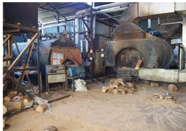
Fuelwood boiler (right) and decommissioned fuel oil boiler (left), Makomboki
