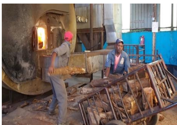
Boiler feeding from handcart, Makomboki
