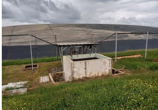
Agitator (recirculation pump) (Francis Kemausuor)
