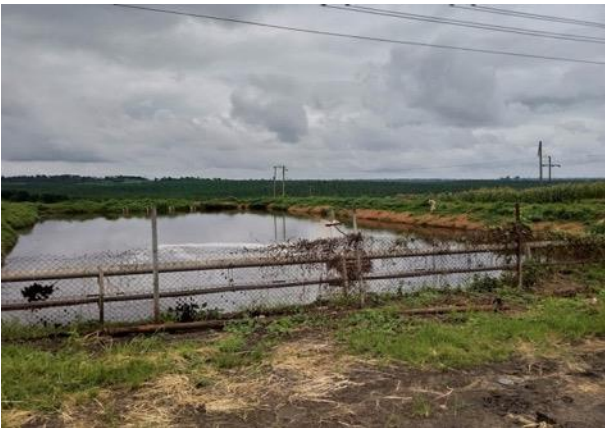
1 st stage digestate pond (Francis Kemausuor)
