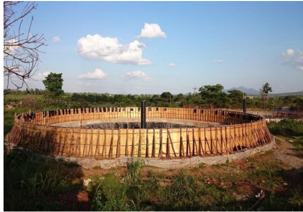
Timber formwork for casting the digester walls (Hannes Muntingh)
