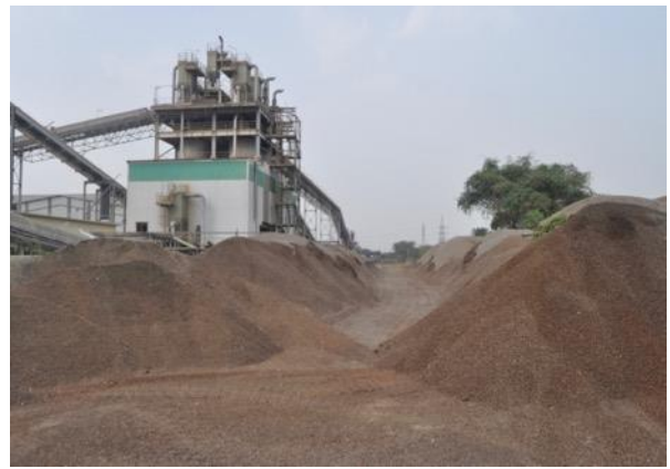
PKS storage at Ewekoro II
