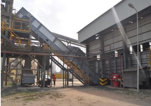
Lift from walking floor to magnetic separator, Ewekoro II
